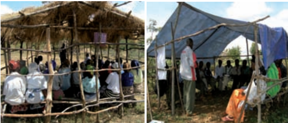
Temporary Roofing Structure
